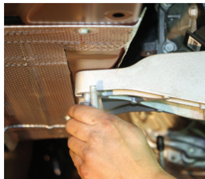
We used a transjack to support the transmission so the crossmember bolts could be removed.
